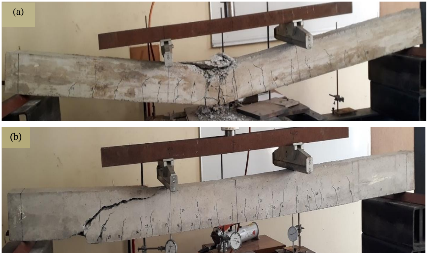
Figure5. Flexural test failure patterns of controlled specimens of RC beam reinforced with (a) M1 and (b) M2 at ultimate failure
