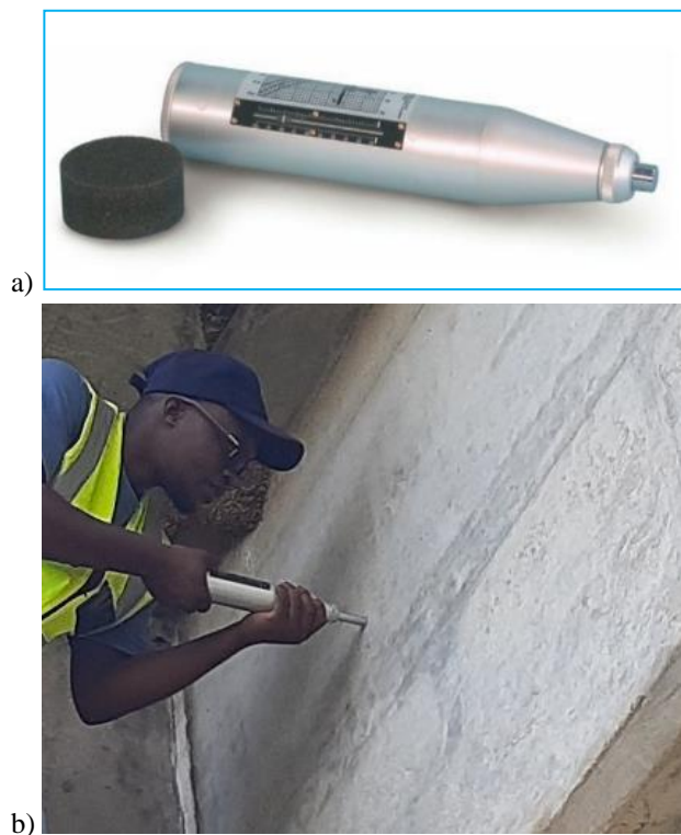
Figure 2. (a) N Type concrete test hammer and (b) on-site test process
