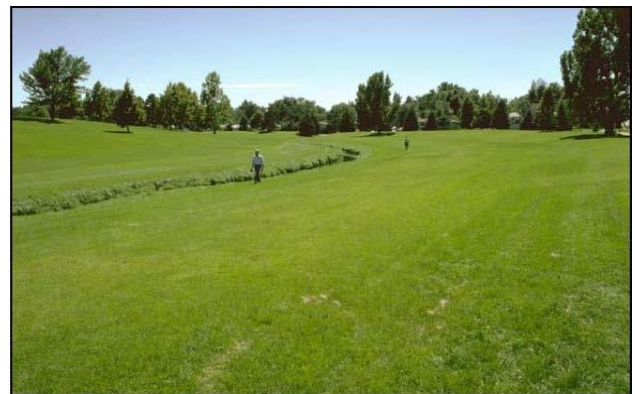
Figure 3. A wide-open waterway carries floodwater at modest depths while maintaining low velocities to inhibit erosion.
