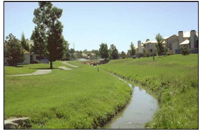
Figure 2. Use of uniform design standards represents a reasonable standard of care for urban flood channels.
