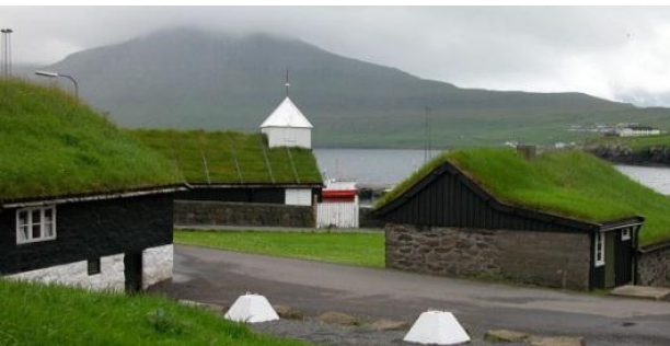
Figure 6. Lawn roofs in rural house in Norway (Brandada, 2007).
