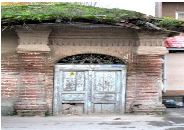
Figure 5. Plant growing on the earthenware coverage of traditional roofs in Mazandaran (writers, 2013).
