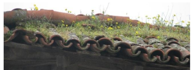
Figure 4. Plant growing on the earthenware cover of traditional roofs in Mazandaran (writers, 2013).
