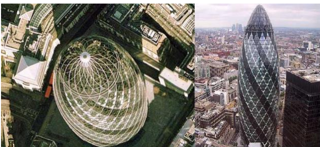
Figure 3. St Mary Axe 30 Tower
