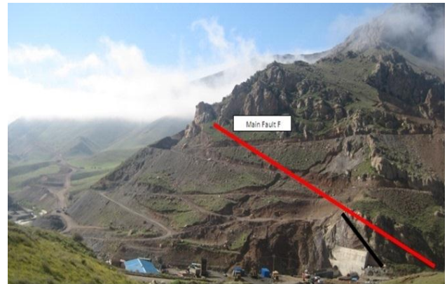
Figure 2. A view of fault f from outlet of tunnel
