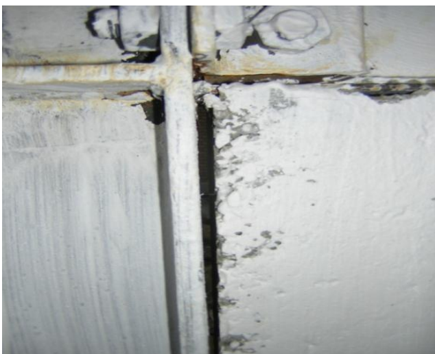
Figure 6. Boundary separation in the corner of the infill
