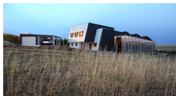
Figure 1. The Use of Natural Elements in Design Can Have an Important Role in Reducing Energy Consumption (Aldinga Arts Eco Village Sustainable House, Aldinga, South Australia).
