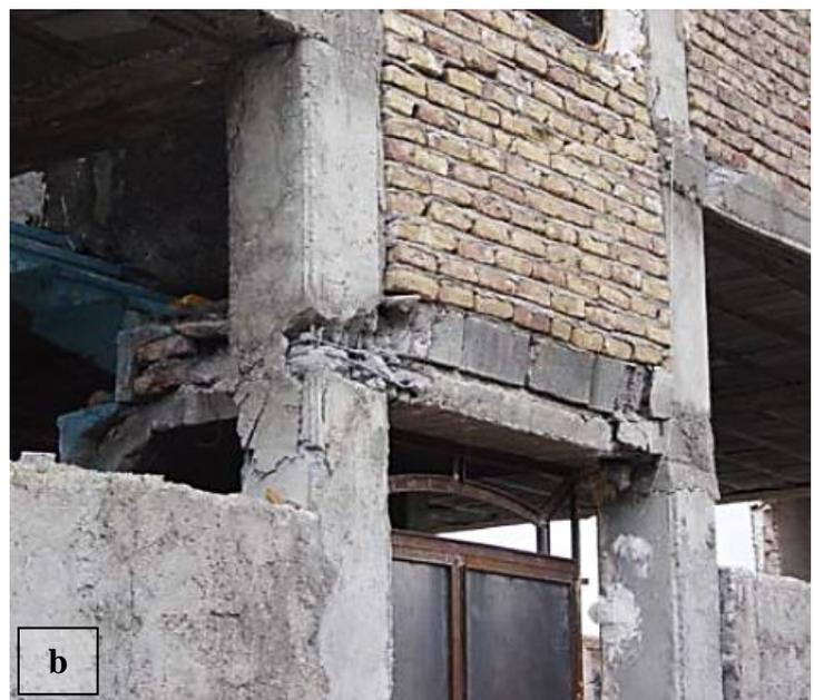
**Figure 8.** Stairway-Frame interaction failure in past earthquakes; (a) 2010 Chile Earthquake stairway bracing action failure (FEMA E-74, 2011), (b) 2003 Bam Earthquake stairway short column failure (Vaseghi, 2003).
