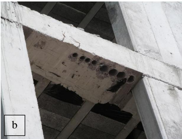
**Figure 15.** Five-story building with unacceptable pipe passing detail; (a) overall view, (b) beam-shear wall connection detail
