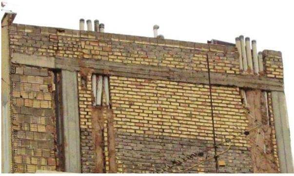
**Figure 14.** Wrong pipe and sleeve passing through high bending moment zones
