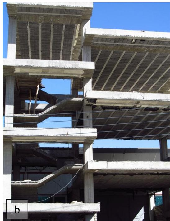
**Figure 16.** Stairway-Frame interaction failure potentialities; (a) building view, (b) detail view
