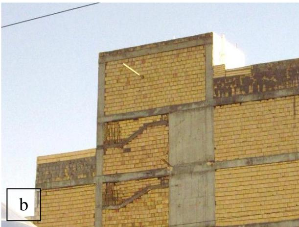
**Figure 17.** Two buildings in Esfahan with high risk of brittle stairway and short column failure
