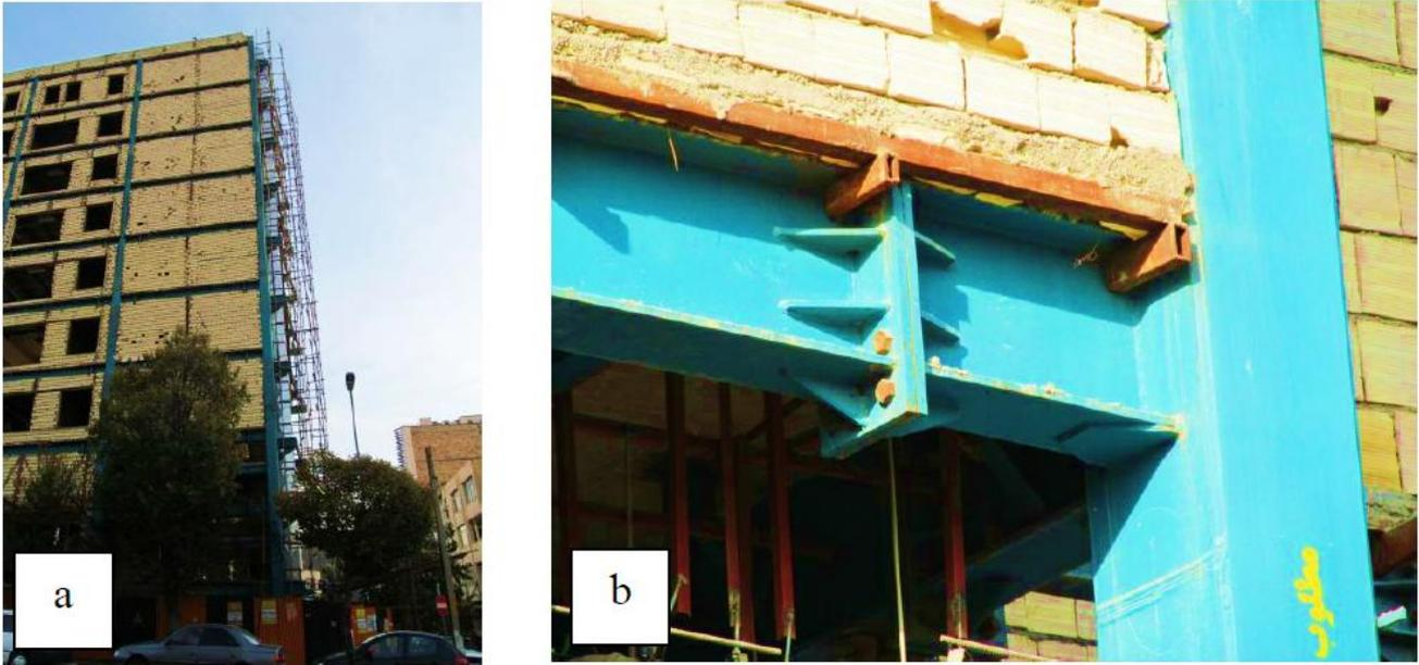
**Figure 9.** Ten-story Steel structural with protected zone imperfection; (a) building elevation, (b) beam-column view
