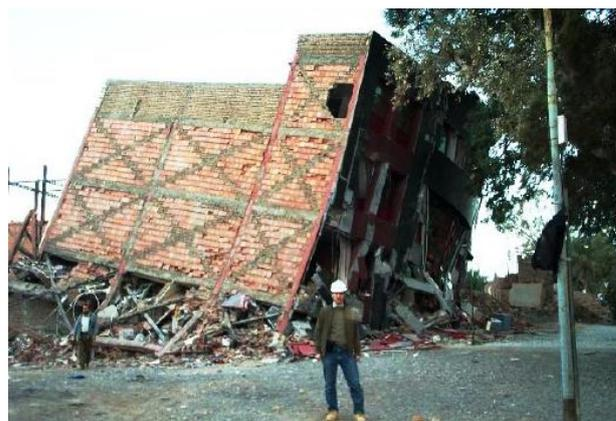
Figure 1. Steel structure failure in Bam (Manafpour, 2008)
