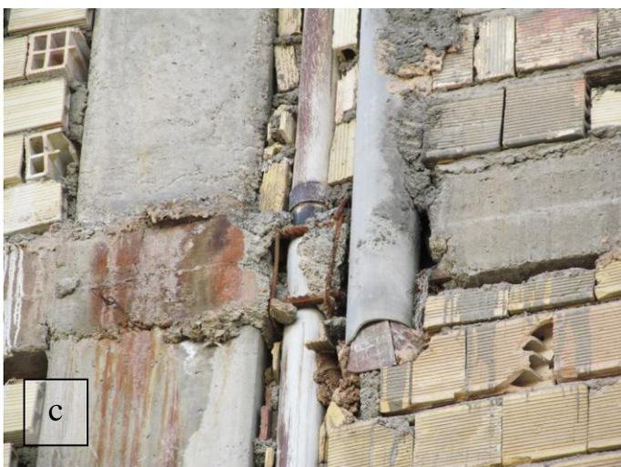
**Figure 13.** Wrong pipe and sleeve passing through cantilever beam; (a) Building North elevation, (b) Building East elevation, (c) detail A- Beam to column connection detail
