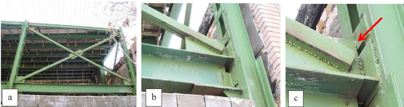
**Figure 11.** Two-story Steel structural with tie plate imperfection; (a) building elevation, (b) beam-column view, (c) detail view of connection
