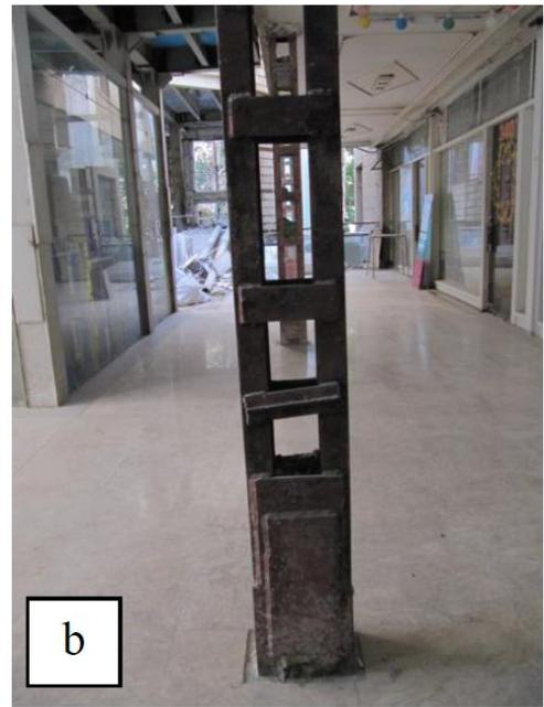
**Figure 12.** Two buildings with constructional defects; (a) Incorrect usages of tie plates, (b) irregular arrangement of lacing plates
