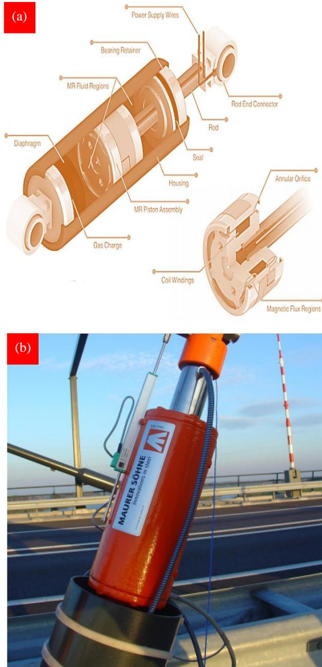
**Figure 10.** Implementation of MR dampers in structural control of a bridge: (a) the detailed 3D schematic of the prototype; (b) the photograph of the damper right after installation (Weber et al., 2006)
